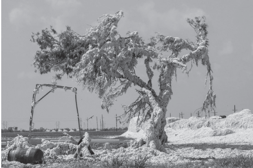
Hurricane Harvey severely damaged the Bayside-Richardson Cotton Gin facility in Woodsboro, Texas, in 2017. Lance Cheung/USDA.
